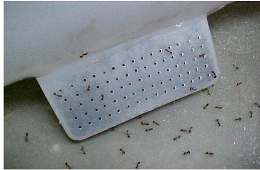
**Fig. 2.** Worker ants escaping weep hole cover.
